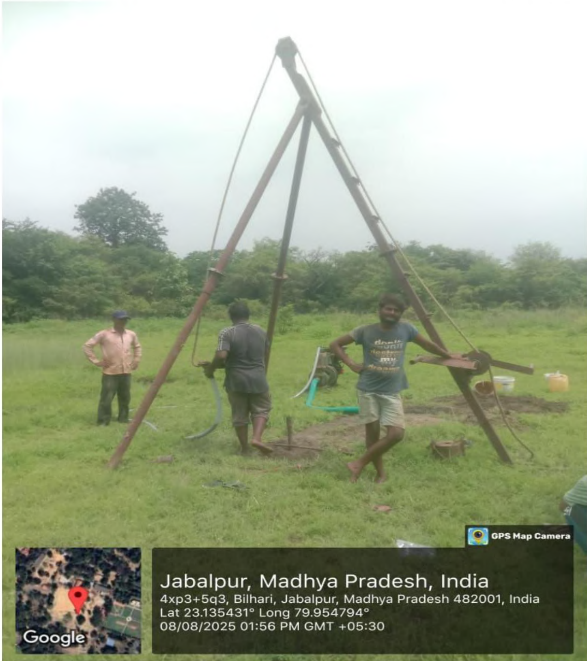
SOIL INVESTIGATION WORK AT DIFFERENT LOCATION AT JABALPUR, MADHYA PRADESH
