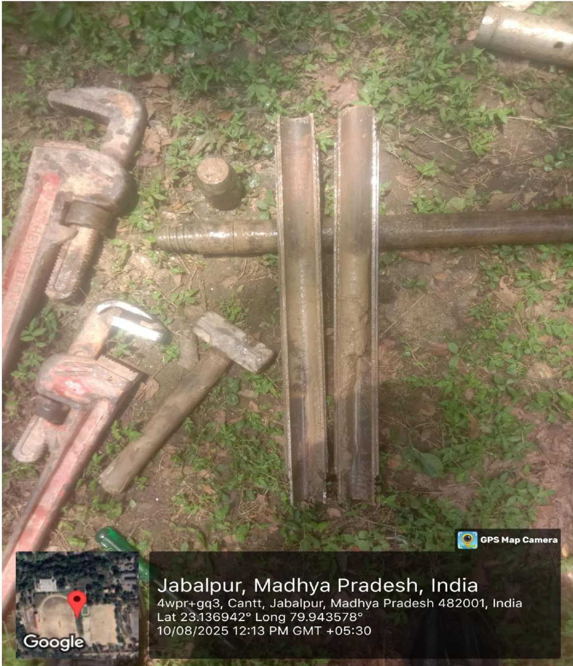
SOIL INVESTIGATION WORK AT DIFFERENT LOCATION AT JABALPUR, MADHYA PRADESH
